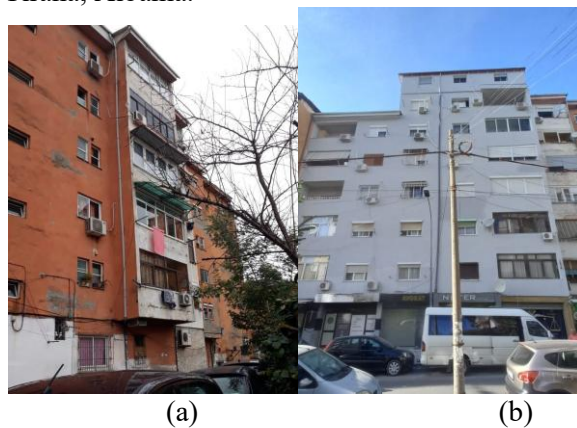
Figure 2. 'Haxhi Hysen Dalli' road, (a) before and (b) after façade renovation
