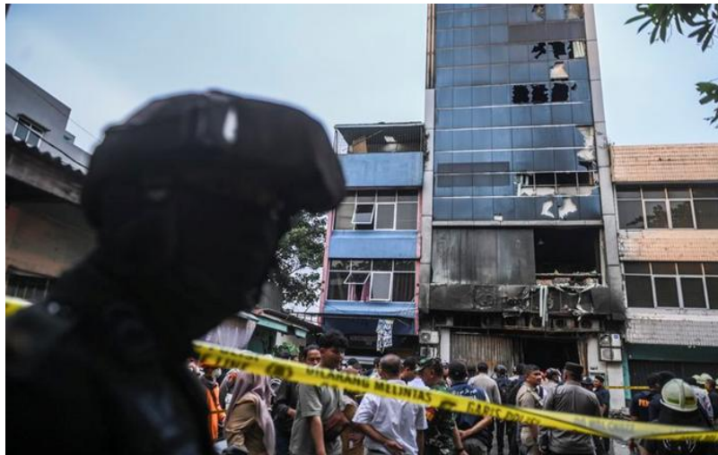
Figure 1. Terra Drone Building Fire Incident
