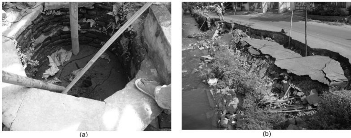
Figure 1. Liquefaction phenomena observed during the 2006 Yogyakarta earthquake: (a) sand boils, (b) lateral spreading (Maze, 2017)
